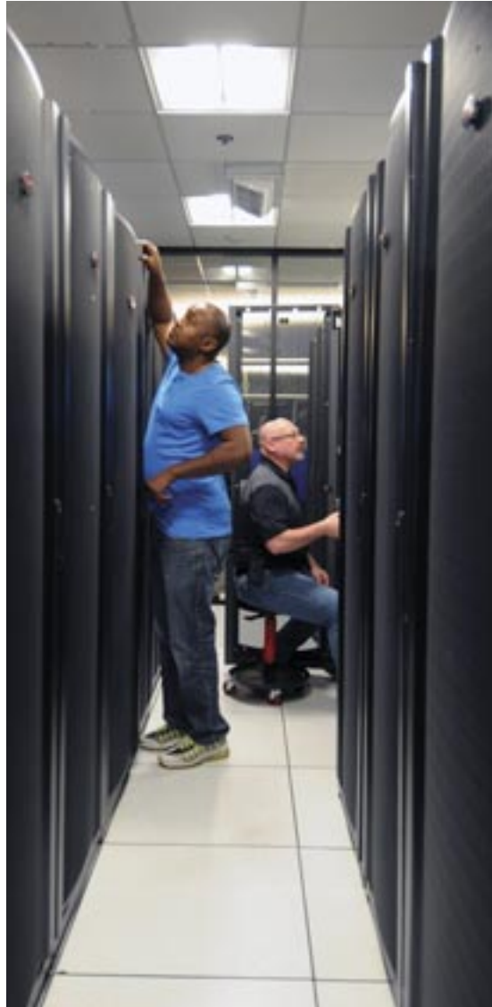
Part of the APS computer room, where servers for the electron storage ring and x-ray beamlines are located.
